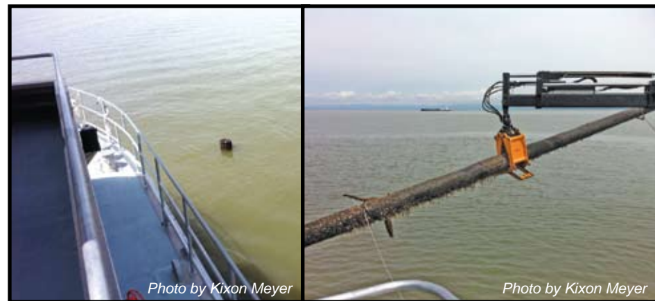
A “deadhead” is a large wooden post or tree that hangs vertically in the water with only the top exposed (left). Only after the crew worked this obstacle loose from the muddy bottom and removed it could the actual size of the hazard be seen (right).
