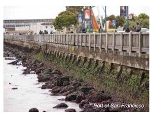
The Seawall is essentially a rock retaining wall built before modern engineering techniques to address earthquakes.
