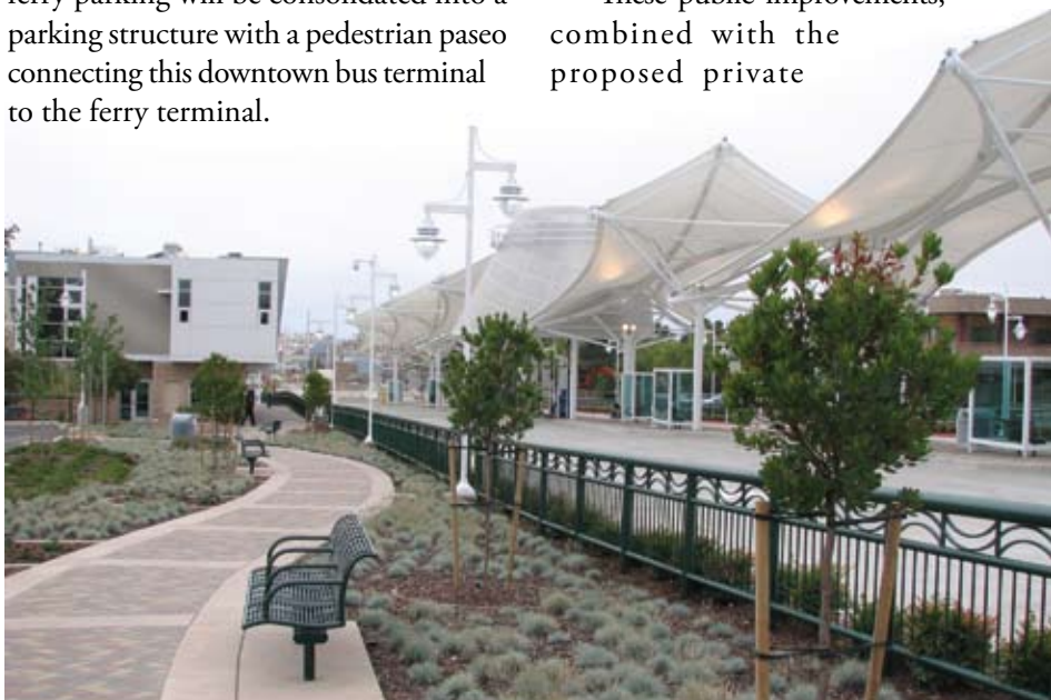
The Vallejo Transit Center represents the first major step toward the transit-oriented development envisioned in the City's specific plans for its waterfront and downtown.
