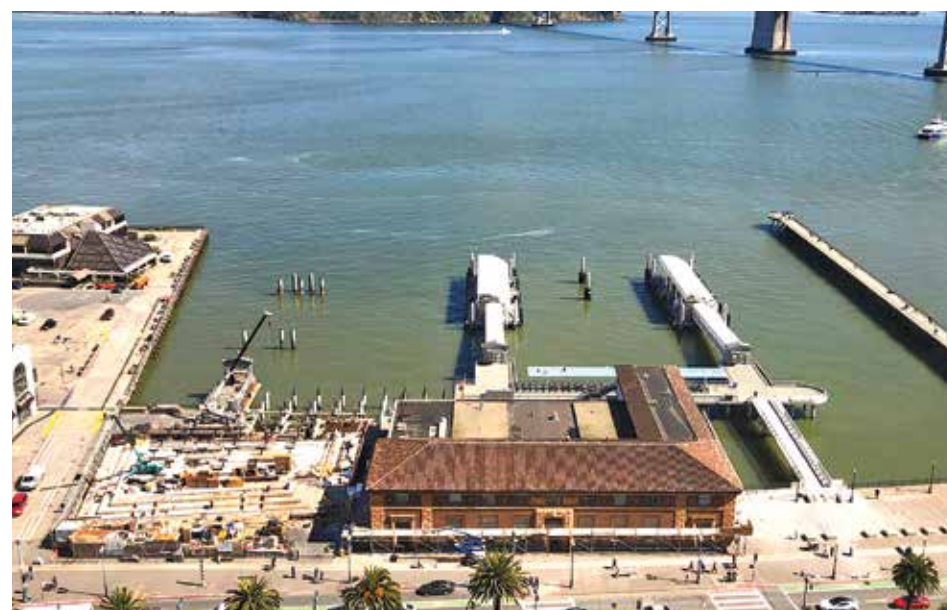
WETA Downtown San Francisco Ferry Terminal Expansion, March 2019
