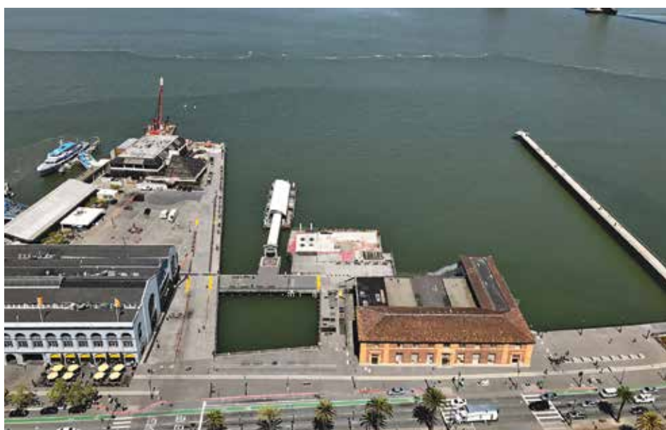
WETA Downtown San Francisco Ferry Terminal Expansion, June 2017
