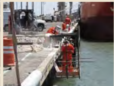
Chevron Long Wharf Marine Engineering Construction
