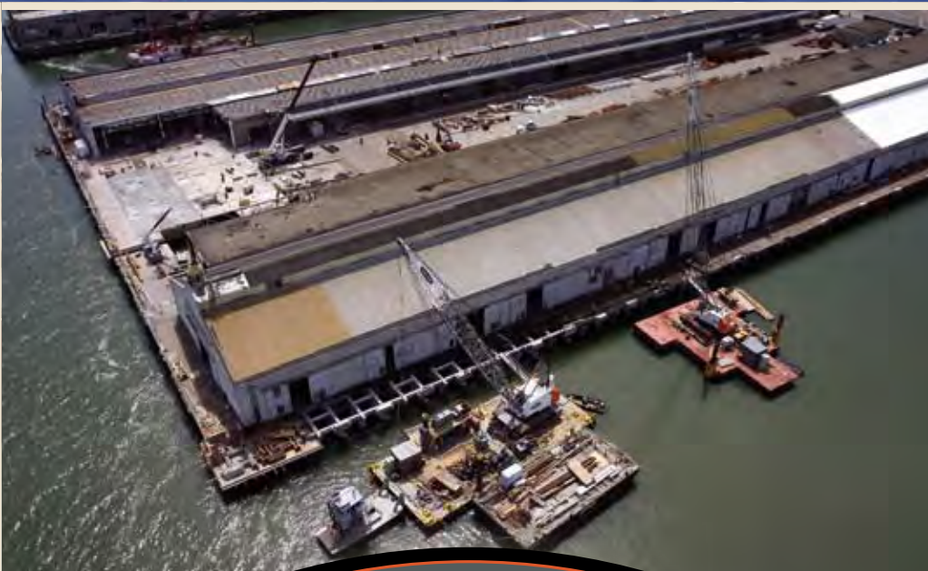
Exploratorium Museum at Pier 15
