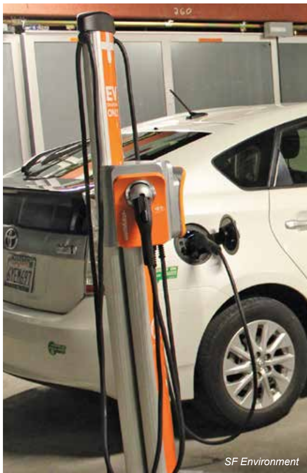
In January, new buildings in San Francisco must be outfitted with sufficient electrical infrastructure to simultaneously charge electric vehicles in 10 to 20 percent of on-property parking spaces.
