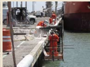
Chevron Long Wharf Marine Engineering Construction
