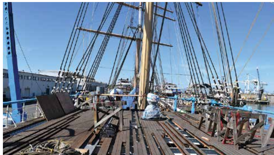
Repairs being made include the replacement of many of the wood planks on the poop deck.
