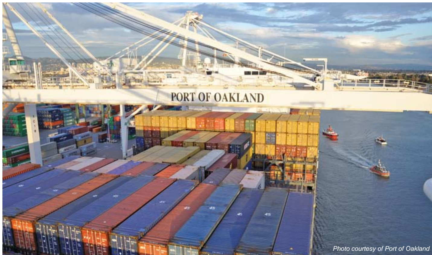
Photo courtesy of Port of Oakland As of last November, the large cranes used at the Port of Oakland to offload containers from vessels run on electricity from the port's recently completed shore-to-ship power grid.
