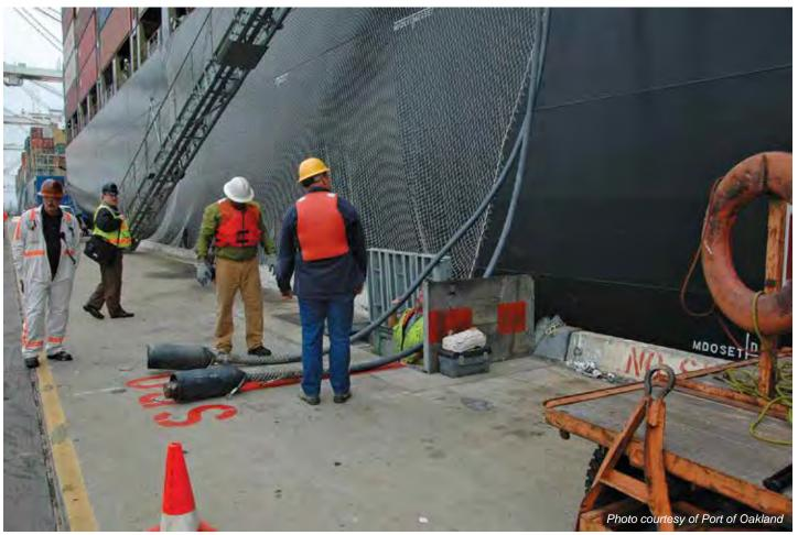
Since 2012, vessels docked at the Port of Oakland have been able to switch off their diesel-powered engines and plug into an on-land electrical grid to keep onboard lighting and equipment operational while berthed.
